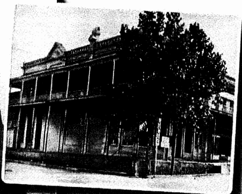
Gibbs National Bank, northeast corner of 11th Street and Sam Houston Ave. The first streets were paved in 1918.
